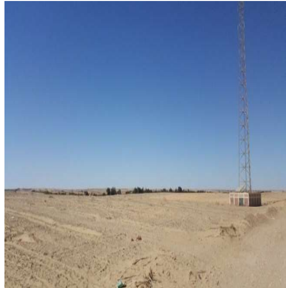
Figure (4-2): Southern side of the TS.
